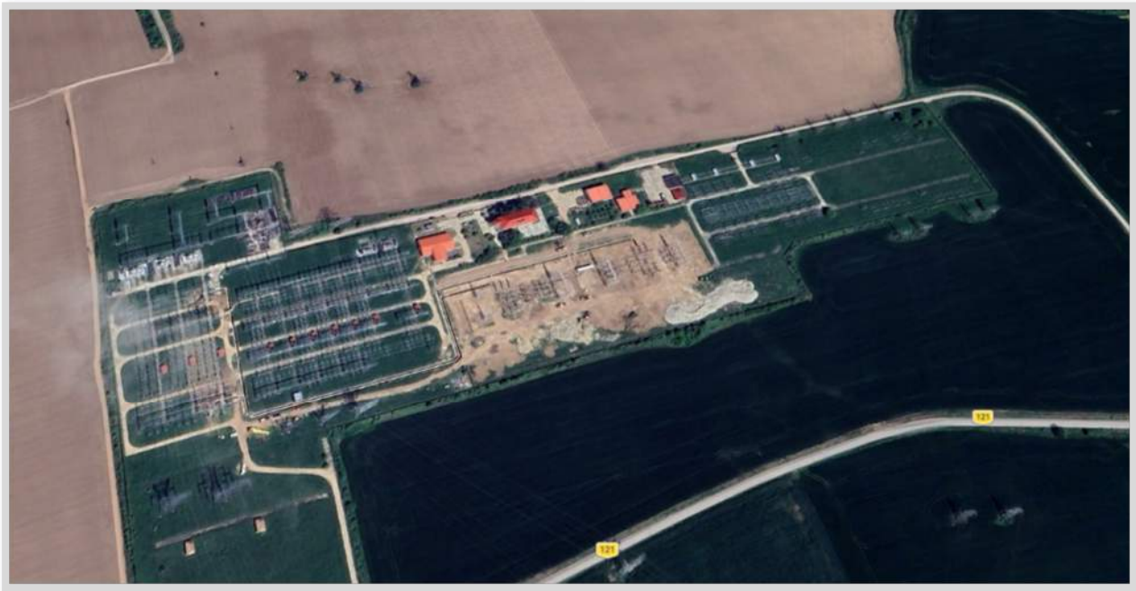
Figure 4-2 400/220/110 kV Gutinaș Substation
